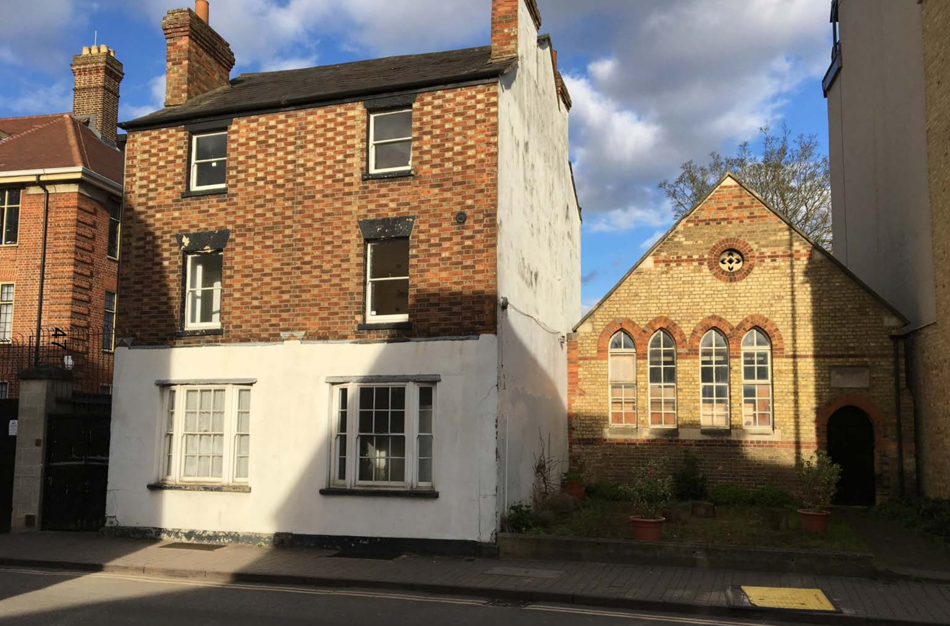
View of 120-121 Walton Street with Bedford House alongside and set back from the frontage
